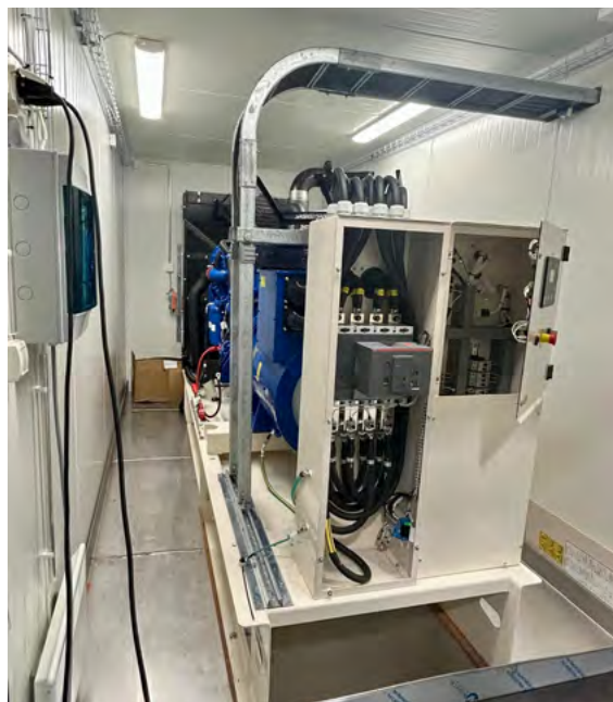
Figure 1. Emergency generator built into a sea container
