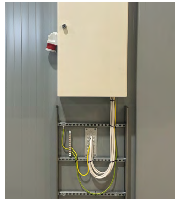
Figure 2. Ready-made connection point for an emergency generator
